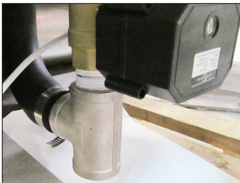
Fig. 5 - Drain valve
